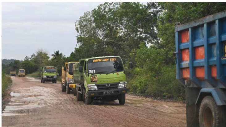
Figure 30. Trucks transporting landfill to the construction site of PT Phoenix International Resources in December 2022.
