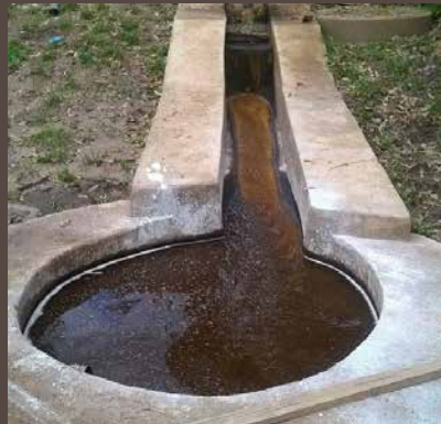
Neutralization tank, part of the wastewater treatment system at the Sovu coffee washing station.
