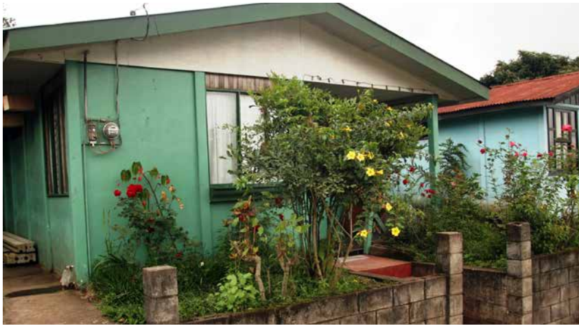
Worker housing on the Aquiares coffee farm in Costa Rica.
